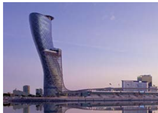
Hyatt Capital Gate Hotel, Abu Dhabi. Hansgrohe products: Raindance S 240 Air overhead shower. Photo: abudhabi.capitalgate.hyatt.com
