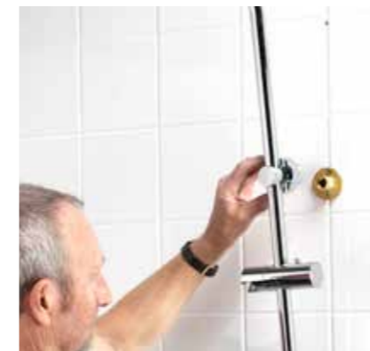
4 Secure valve & connect to the existing pipe fittings
