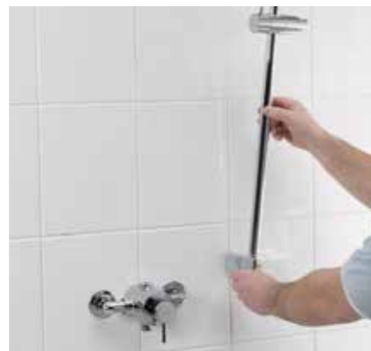
5 Fit the rail system to wall, and attach the head & hose
