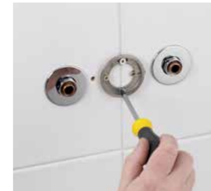
2 Remove mounting plate & fit the Aspire mounting plate
