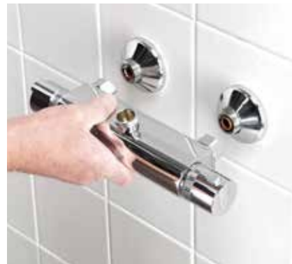
1 Remove the shower system from the wall leaving the valve fittings if required
