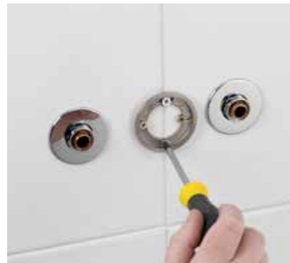
2 Remove mounting plate & fit the Siren mounting plate
