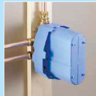
1. Fix the mixer body into position and connect the pipework.
