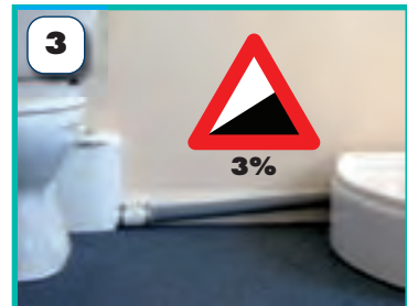
Where the pipework falls to a floor lower for example, fit an air admittance valve at the highest point capable of withstanding 10psi pressure, or increase pipe size coming down to 'break' syphon.
