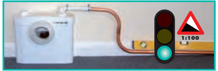
Discharge pipework should be copper or rigid solvent weld plastic, not 'pushfit'
