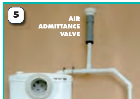
Where the pipework falls to a floor lower for example, fit an air admittance valve at the highest point capable of withstanding 10psi pressure, or increase pipe size coming down to 'break' syphon.
