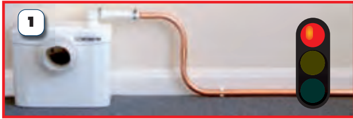
All horizontal pipes should have a minimum fall of 1:100.
